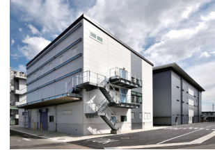
Polymer pilot plant building
