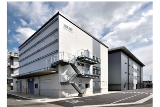
Polymer pilot plant building
