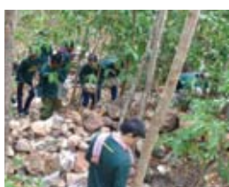
Check dam installation
