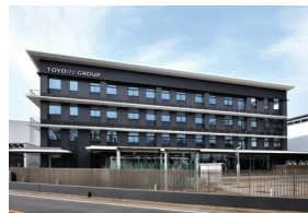
The new Technical & Administration Building at Kawagoe Factory
